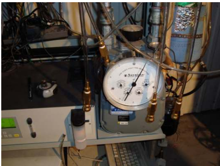
Picture 8: Reference dry gas meter
